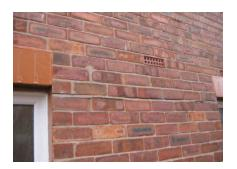
2. Horizontal cracking. A sign of wall tie failure. A common fault in older properties where the ties corrode. If your home is showing similar symptoms act sooner rather than later.
