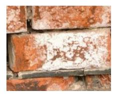
**5.**Efflorescence is the deposit of soluble salts left on bricks when the water in which they were dissolved evaporates. Most efflorescence is harmless, though it has an unattractive appearance. As efflorescence normally affects new buildings in the first three months, it is best left to weather away by itself. Although efflorescence can be removed manually, this may cause an unsatisfactory appearance.
