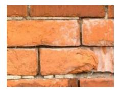
**4.** Sulfate attack actually affects mortar and not brickwork. It is however rare, but can be expensive to cure.
